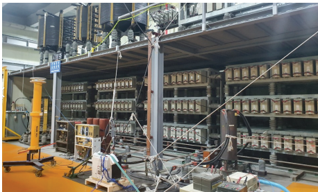
Fig. 4. Simple synthetic test facility.
