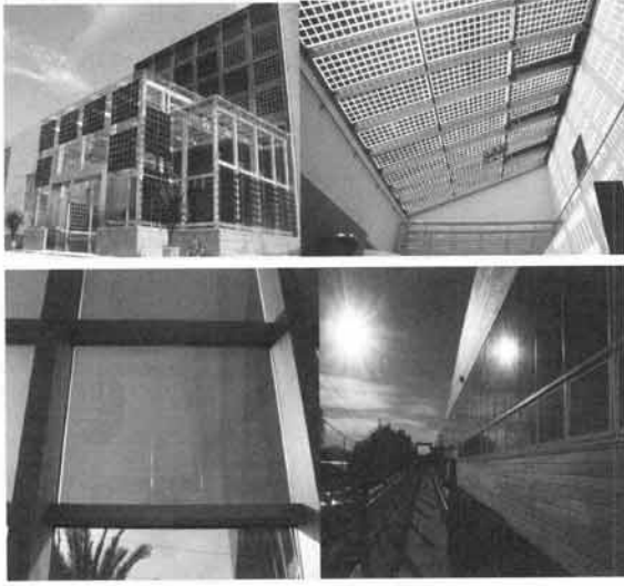
Fig. 4. BiPV systems for building window application.
