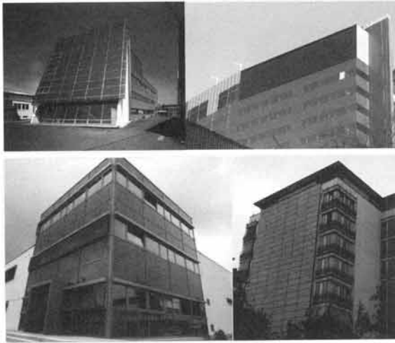
Fig. 5. Wall integration PV systems.
