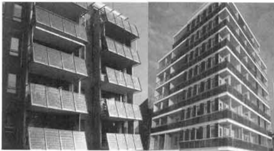
Fig. 8. BiPV systems for balcony.
